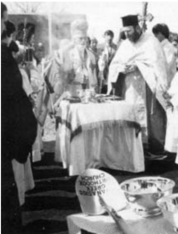
Groundbreaking of the Church
