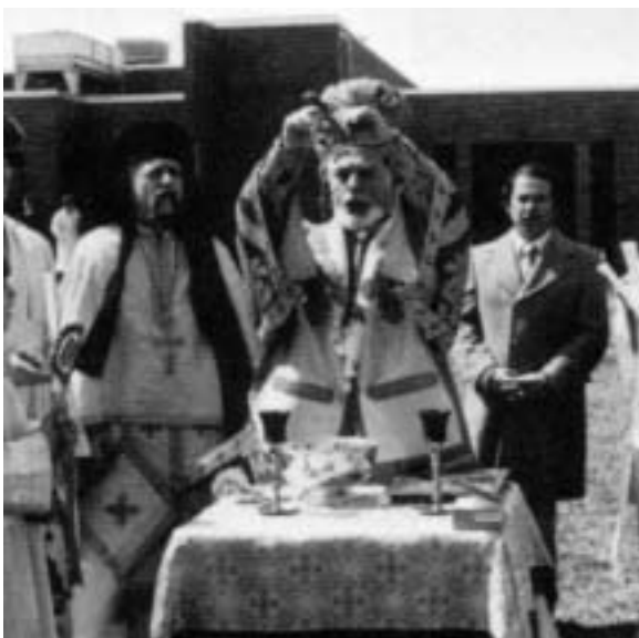
Groundbreaking of the Church
