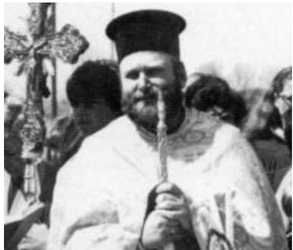
Groundbreaking of the Church
